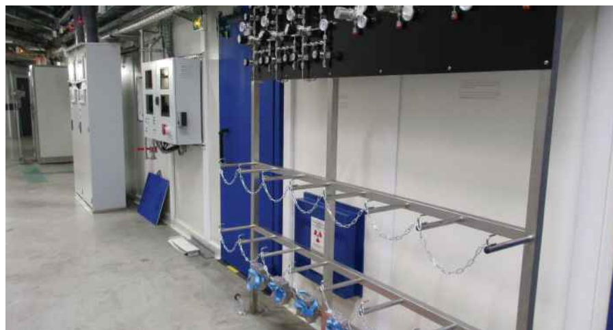
Fig. 4: New gas handling system to keep all the gas bottles for sample environment and ionisation chambers outside the experimental hutch.
